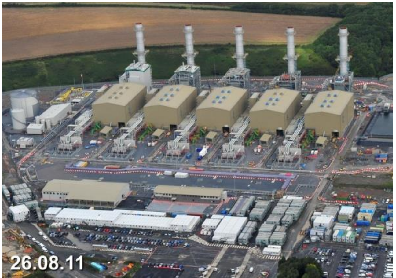
Figure 2 – Image of the Pembroke Combined Cycle Power Plant
